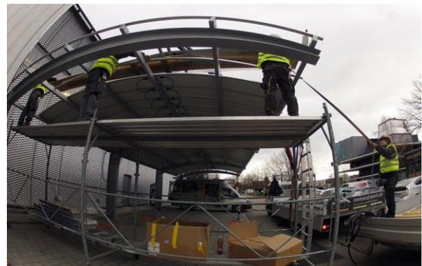
EKZ carport half covered with panels during the installation works
